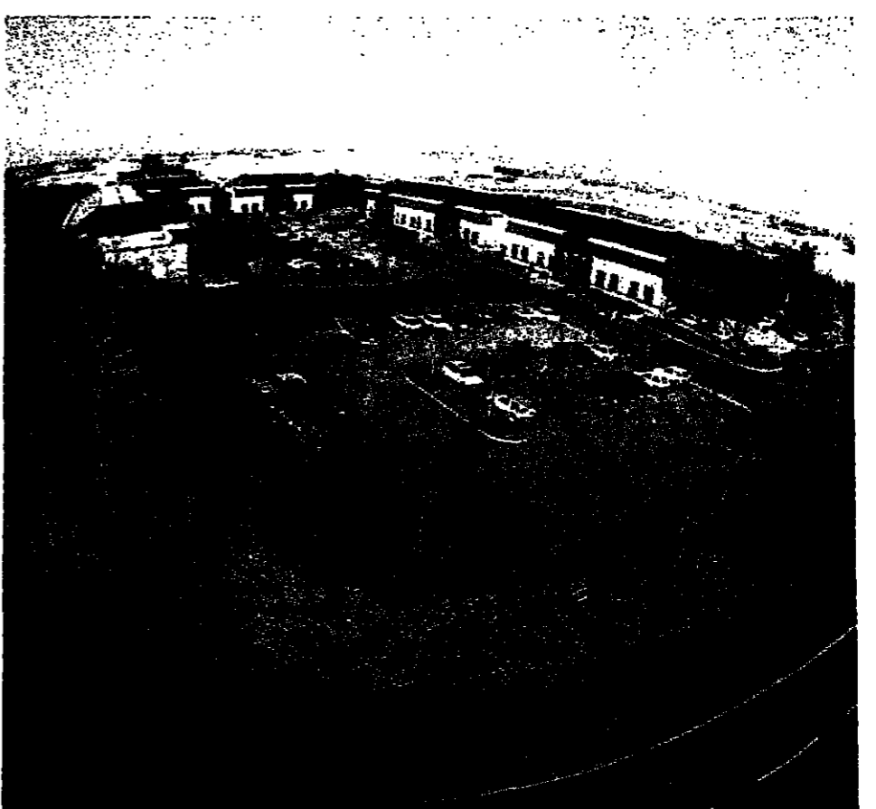
A panoramic view of Gillingham Business Park, Kent. Construction of this park, which was claimed as a first, began in 1978 on the site of a 120-acre disused military barracks
